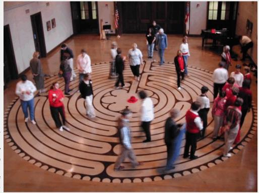
concrete. The cuts of the scoring (photo, top right) give a sharp edge to define the stained area. The stain was a new soy water-based stain which was brushed on in such a way as to give the dark brown lines faux walnut "grain" to match the surrounding extensive woodwork. The different floor colors were achieved by using two different kinds of sealers, one water-based (the labyrinth) and the other solvent-based (the floor).
